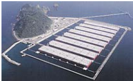
Oil Stockpiling Facility
